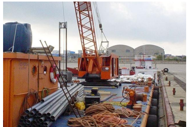
From a barge or multi-cat using big crane.
